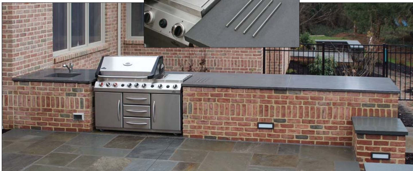
A perfect application for high performance concrete are outdoor kitchens. Integral sinks are one-of-a-kind as are meld basins with countertops. This fusion creates tops that are both sleek and elegant. Built-in trivets can be stainless steel (shown) copper, or brass—providing both a built-in hot plate and a decorative accent. Designer: F. Mula Architects, LLC., Lancaster PA
