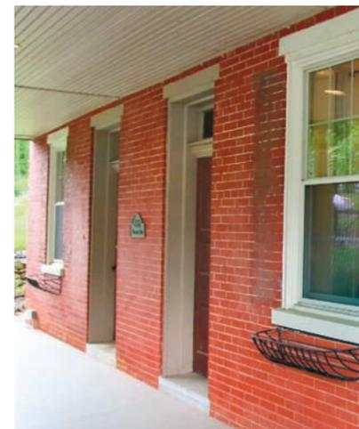
While not changing the exterior appearance, two exterior doors (above) were sealed in the interior to provide additional wall space. In the parlor photo (right), the sealed doors—now wall space—are to the right of the window and, looking into the kitchen, behind the refrigerator.
